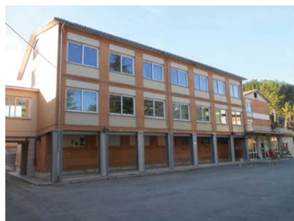
(a) Pilotis at ground floor and strip windows
