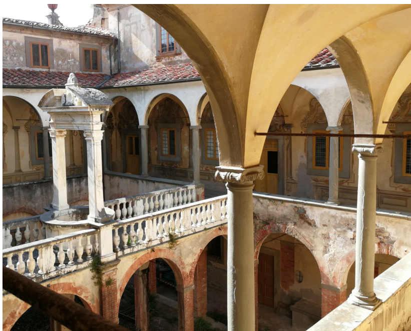
Figure 1. Historic tie-rods: example of tie-rods in one of the internal courtyards in the Certosa di Pisa in Calci, near Pisa, Italy.
