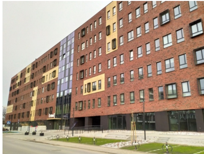
Figure 15. Student Residence Hall Livinn Kraków, renovation and modernisation by Unibep (Item 10, Figure 1) (photo by E. Latusek).
