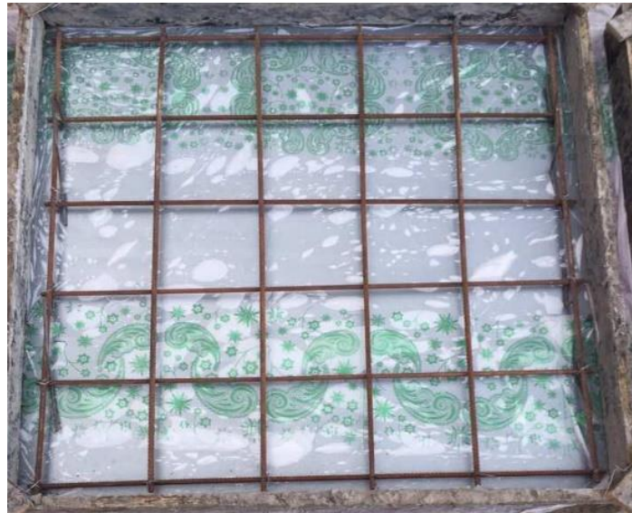
Figure 5. Steel reinforcement and mold.
