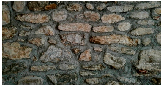
Figure 3. Texture of the masonry.
