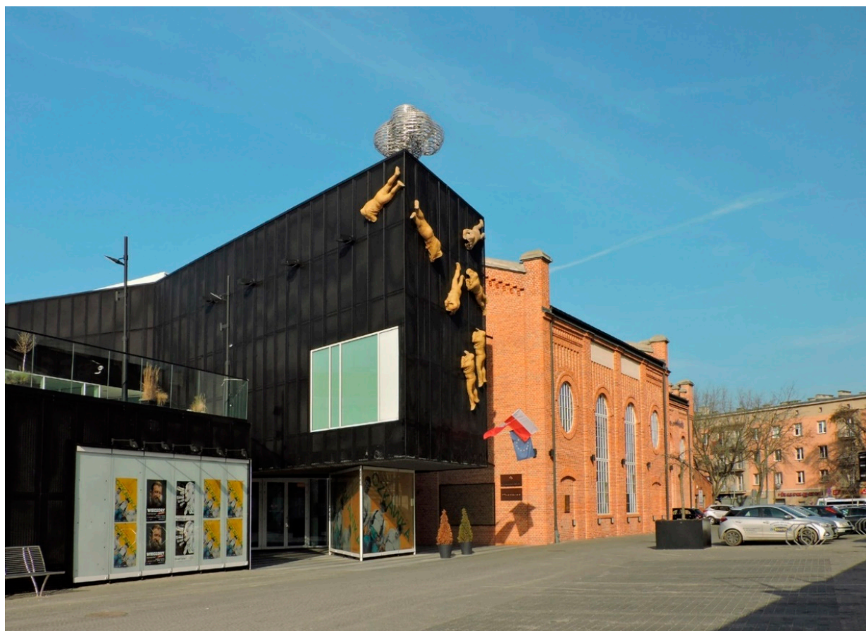
Figure 9. Mazovia Centre for Contemporary Art “Elektrownia” in Radom, photo by Rafał Terkner, Wikimedia Commons, available online: https://upload.wikimedia.org/wikipedia/commons/f/f4/Centrum_Sztuki_Wspolczesnej_Elektrownia_1549766_Fotopolska-Eu.jpg (accessed on 24 September 2021).
