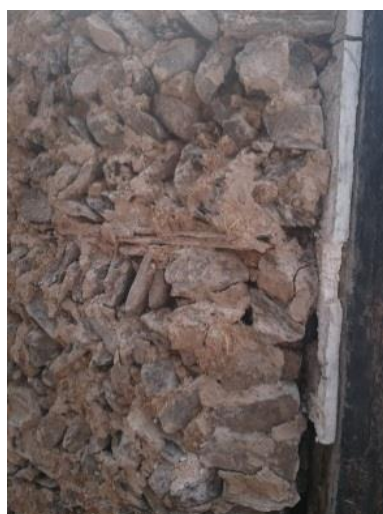
Figure 6. Interface between the timber frame and stone infill.
