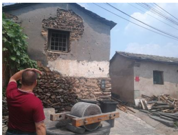
Figure 4. External transverse wall consisting of mud and stone with a window.
