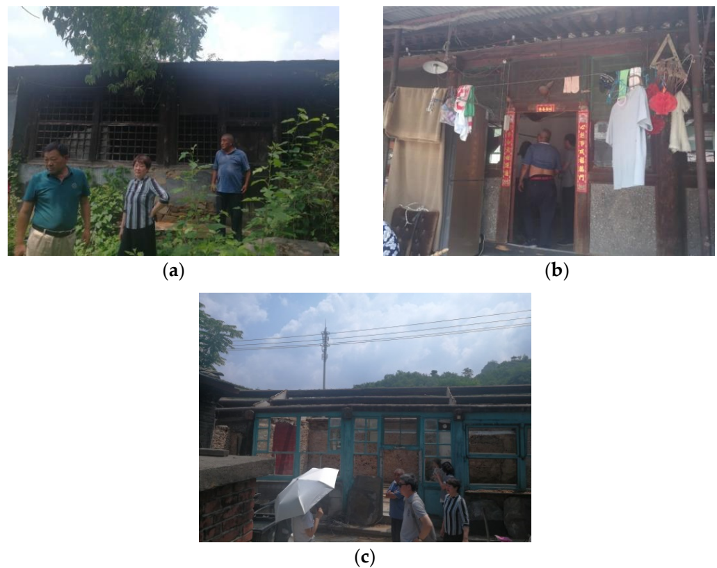
Figure 2. Present situations of traditional residences. (a) Abandoned traditional residence. (b) Traditional residence in use. (c) Repairing a traditional residence.
