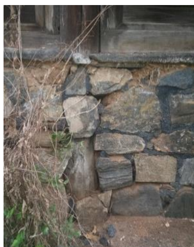
Figure 7. A mixture of mud and straw between the stones.
