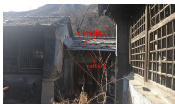
Figure 9. Slate tiles used for roof covering.
