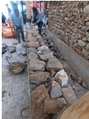
Figure 11. Mud and stone infill construction.
