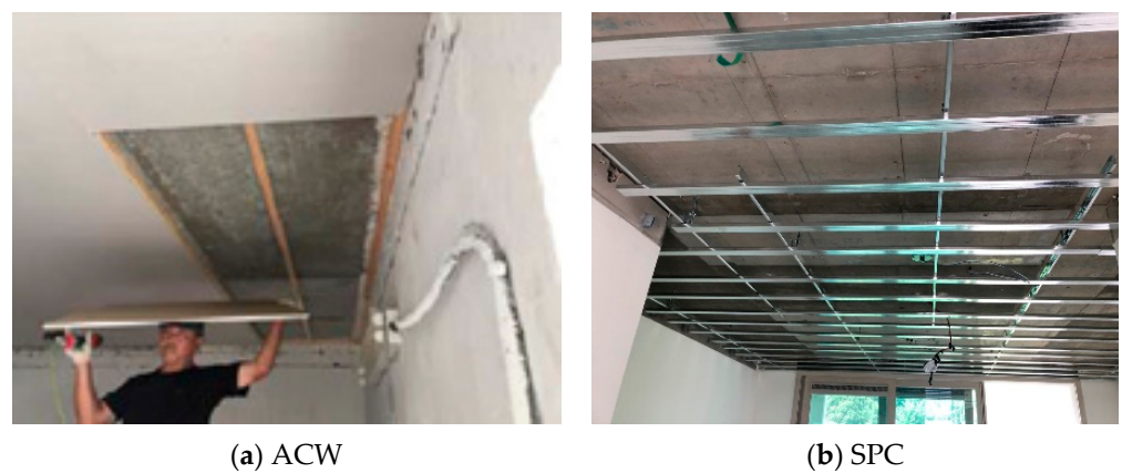
Figure 2. Installation view of conventional ceilings: (a) ACW and (b) SPC.
