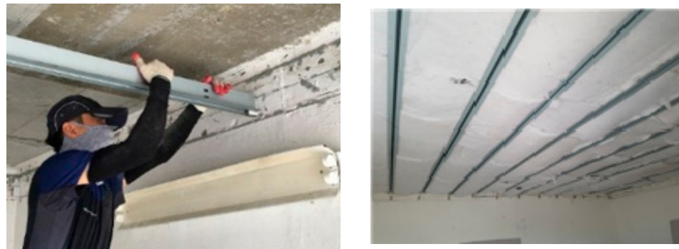
Figure 4. Installation view of the wall-to-wall supported ceiling.
