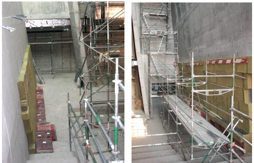
Figure 10. The multi-purpose hall during the acoustic experiment regarding the susceptibility of the room to the formation of the flutter echo. View from the audience on the stage, the left- and right-side walls are shown (photo by A. Kulowski).
