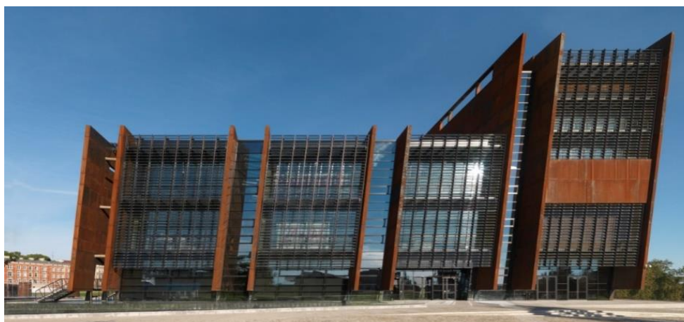
Figure 3. The south and west façade of the ECS, with structural walls which deviate from the vertical by 6.5^\circ . The façades of the ECS are covered with 5 mm thick corten plates (photo by Wojciech Kryński).
