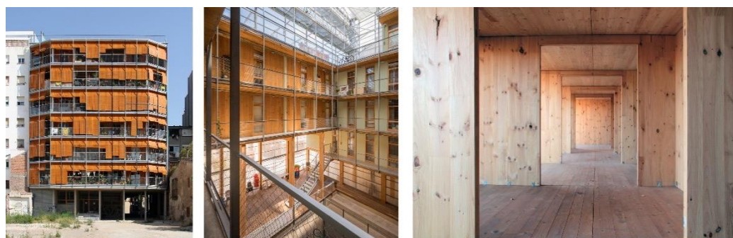
Figure 5. Left: La Borda, housing elevation as seen from Can Batlló. Centre: The courtyard in La Borda forming a central void in the building that connects different uses: bike store (ground floor), large meeting room (1st floor), guest rooms (at the back), dwellings (to the left with a timber facade) and the “greenhouse” rooftop. Right: La Borda under construction. Promenade between dwellings, later enclosed and adapted by the dwellers using “temporary” partitions. Source: Courtesy Lacol (left and right); and Lacol and Lluç Miralles (centre).
