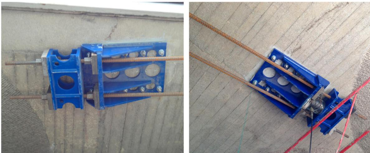
**Figure 22.** Passive (left) and active (right) anchorages.
