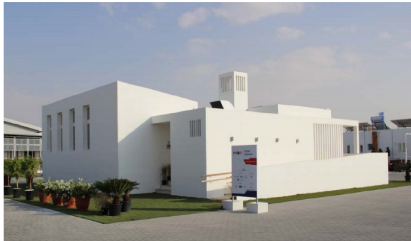
Figure 14. Sapienza house with semitransparent blinds and the wind tower. Reprinted from ref. [70].
