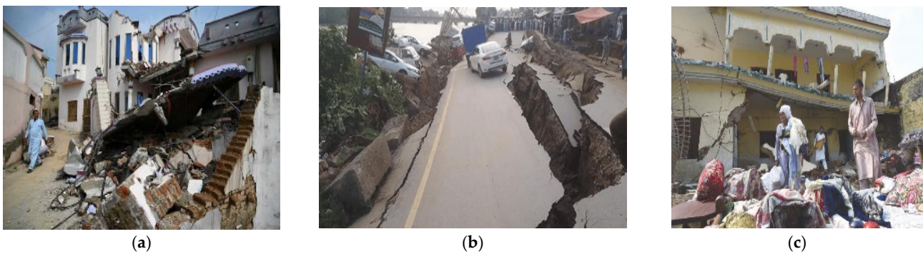
Figure 8. Collapse of RC building (a), damage of road (b), collapse of masonry building (c).
