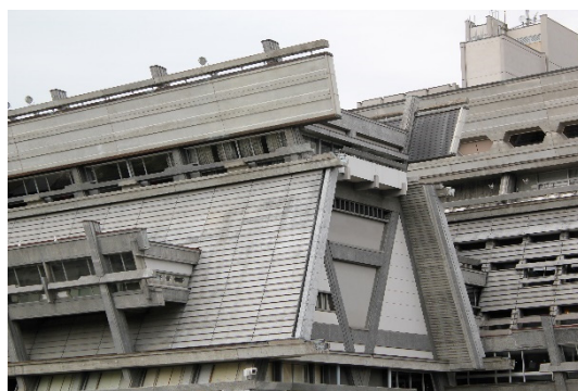
Figure 10. Sachio Otani, Kokusai Kaikan Building in Kyoto, 1963–1966 (photo: Stephen Smith).
