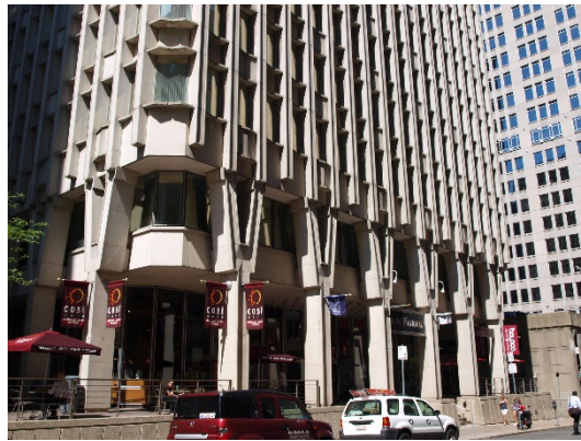
Figure 17. Paul Rudolph, Blue Cross and Blue Shield Building in Boston, 1957–1960 (photo: author of the article).
