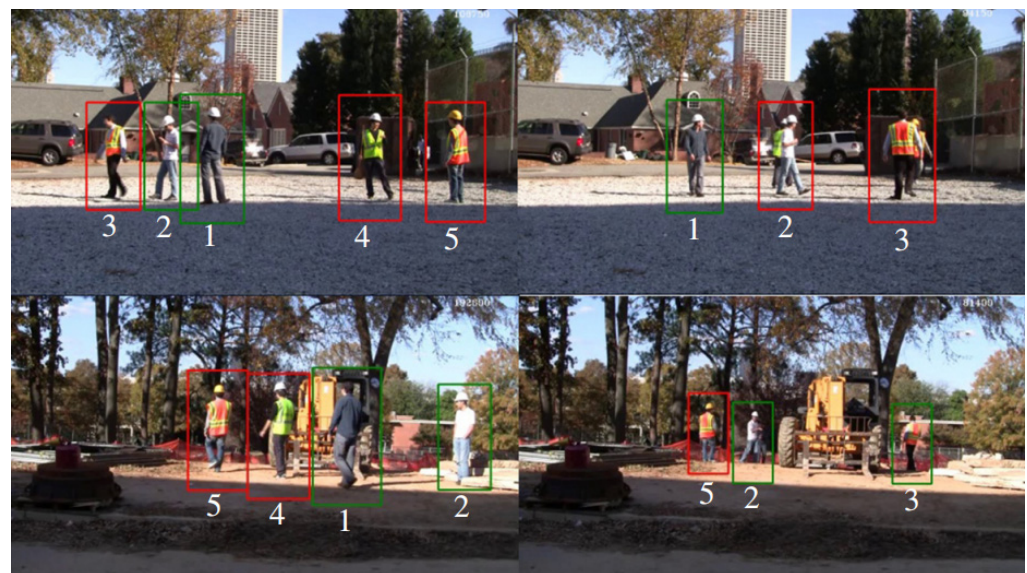
Figure 9. Example of the HOG-based human body detection in the foreground regions. Reproduced with permission from ref. [45]. Copyright 2012 Elsevier.
