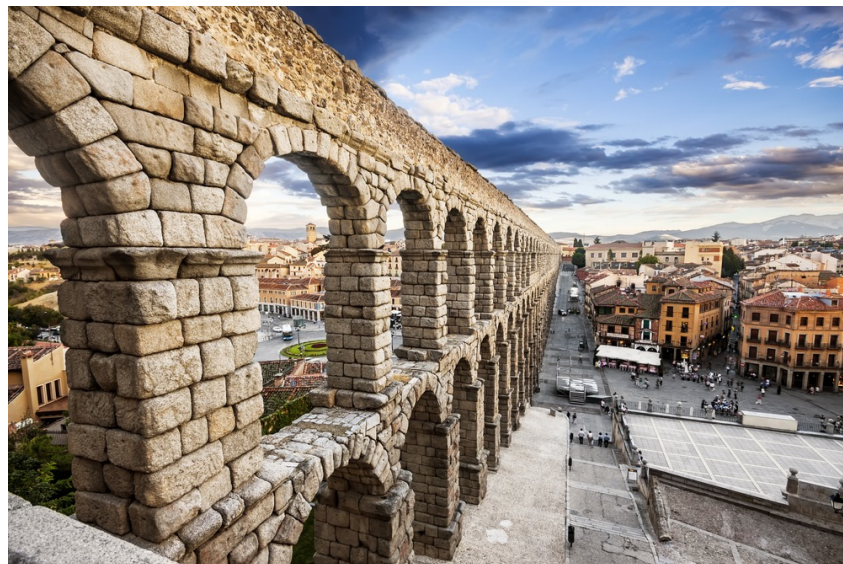
Figure 4. Aqueduct of Segovia (Spain). Granite ashlar without mortar.
