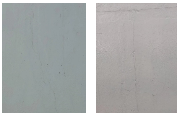
Figure 16. Images of bridge towers.
