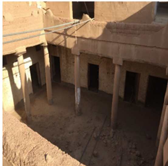
Figure 8. The courtyard shading techniques were used in traditional houses.
