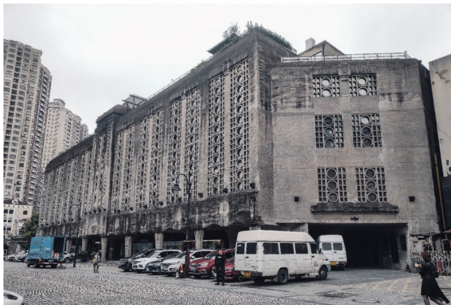
Figure 8. Restored facade of the 1933 Old Millfun (by author 2021).
