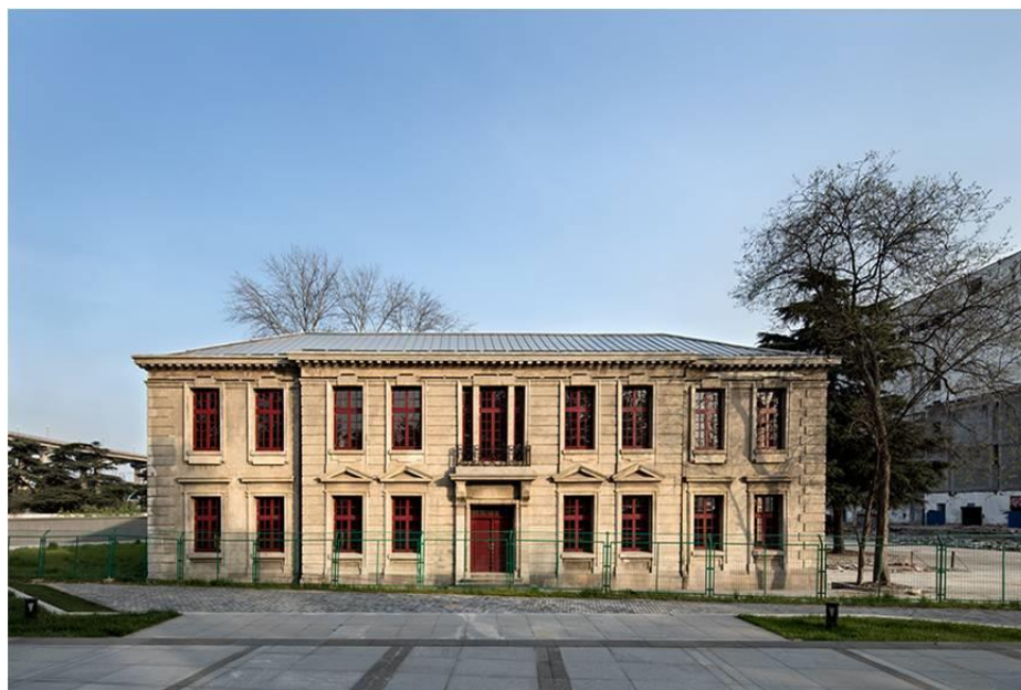
Figure 10. West facade of the Office Building (source: the author's studio).
