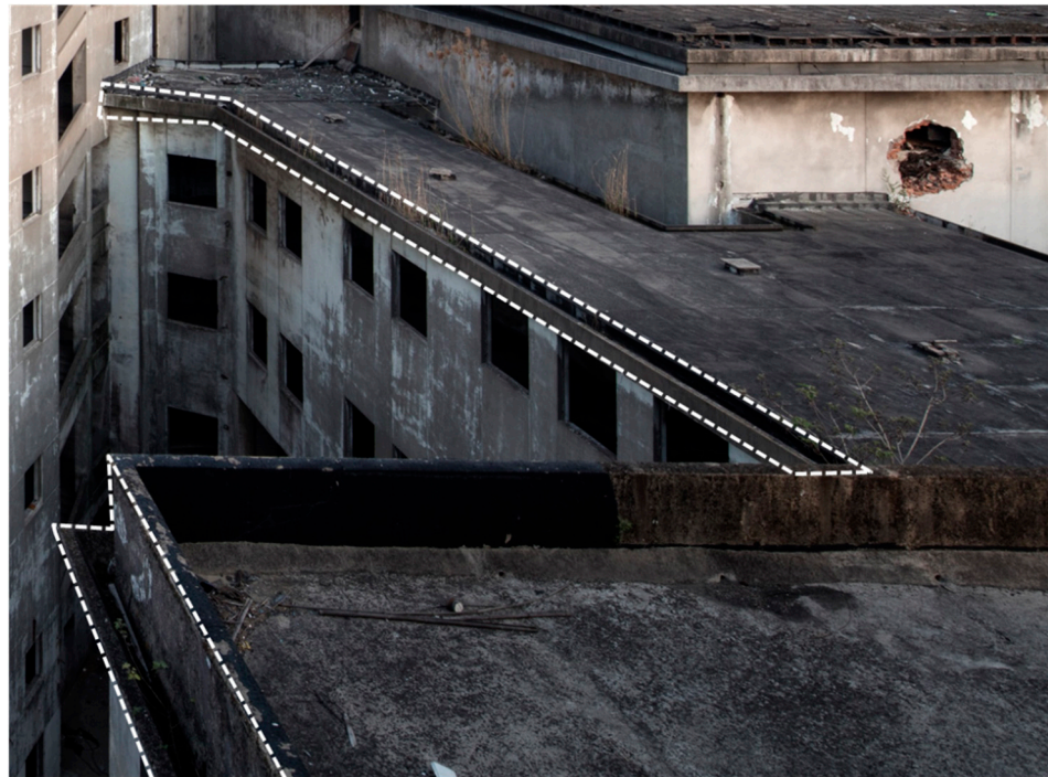
Figure 11. Gutters on the buildings (source: the author's studio).
