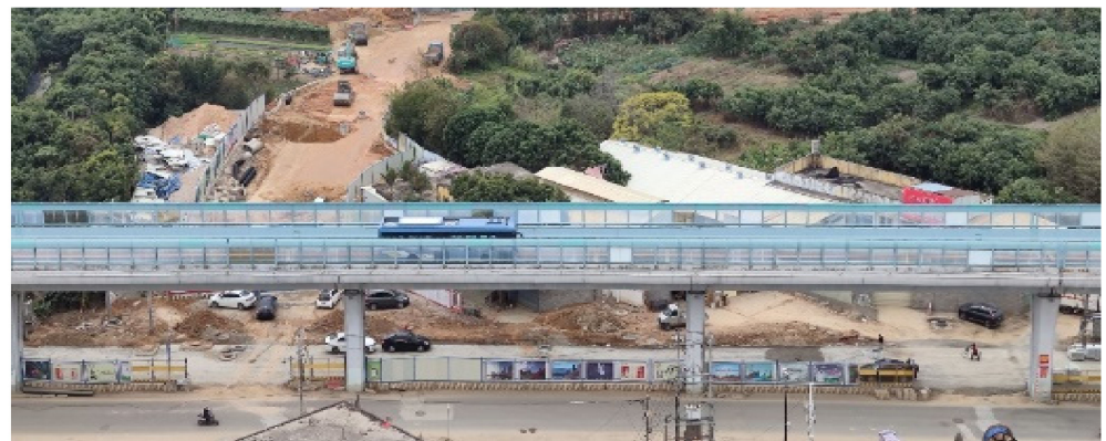
Figure 20. Photo of the BRT Bridge.
