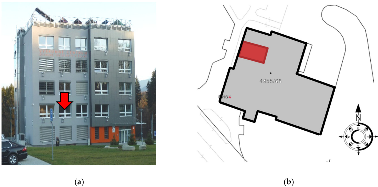
Figure 1. (a) West-side view of the Research Center building with red arrow indicating measured office; (b) floor-plan with red rectangle indicates measured office.
