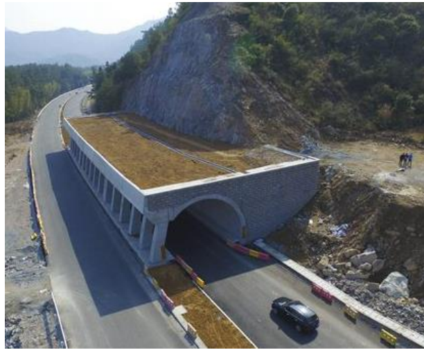
Figure 1. Rock-shed structure applied in actual engineering.
