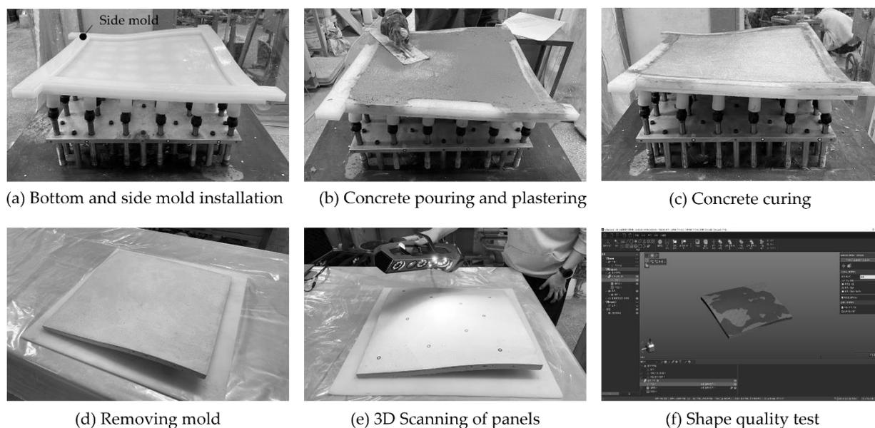
**Figure 12.** Free-form concrete panel fabrication and quality test process.
