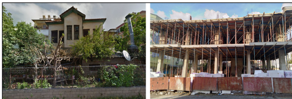
Figure 16. An example of a destroyed and redeveloped historic building in Turkey (It was not listed as a “historic building” before the destruction. The construction started in December 2019).
