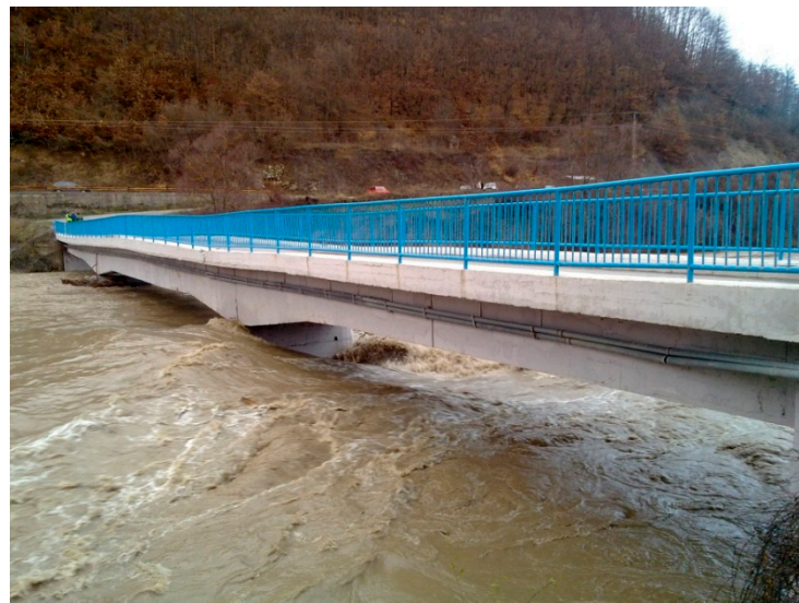
Figure 2. Lim River water level in the area of the Marsenic bridge.
