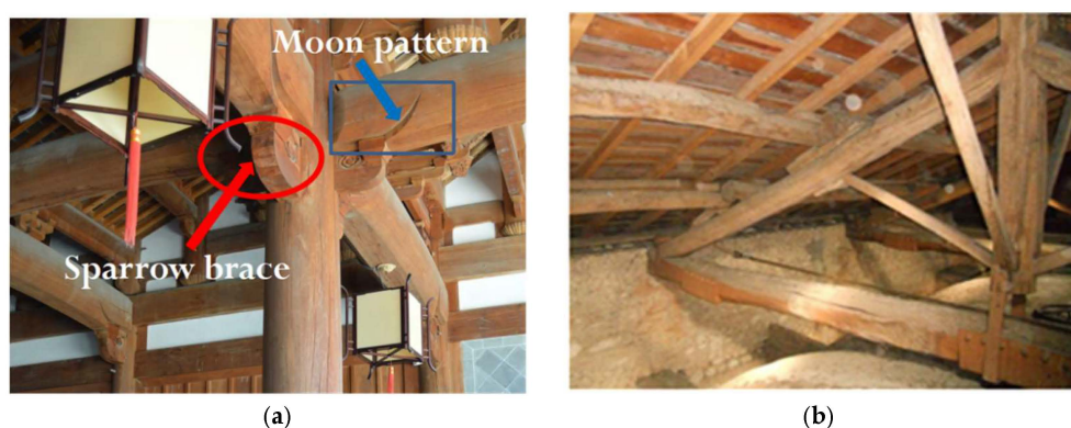
Figure 2. Comparing timber buildings between China and Italy: (a) a folk in Huizhou; (b) a church in Vimercate.
