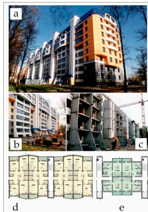
Figure 10. Reconstruction of a house with a superstructure of floors according to project A. Krotov: (a,b) The general view of the house after reconstruction. (c) The reconstruction process. (d,e) Variants of planning solutions, with the organization of a staircase–elevator hall and a change in the apartment. ( https://www.akrotov.ru (accessed on 15 January 2022)).
