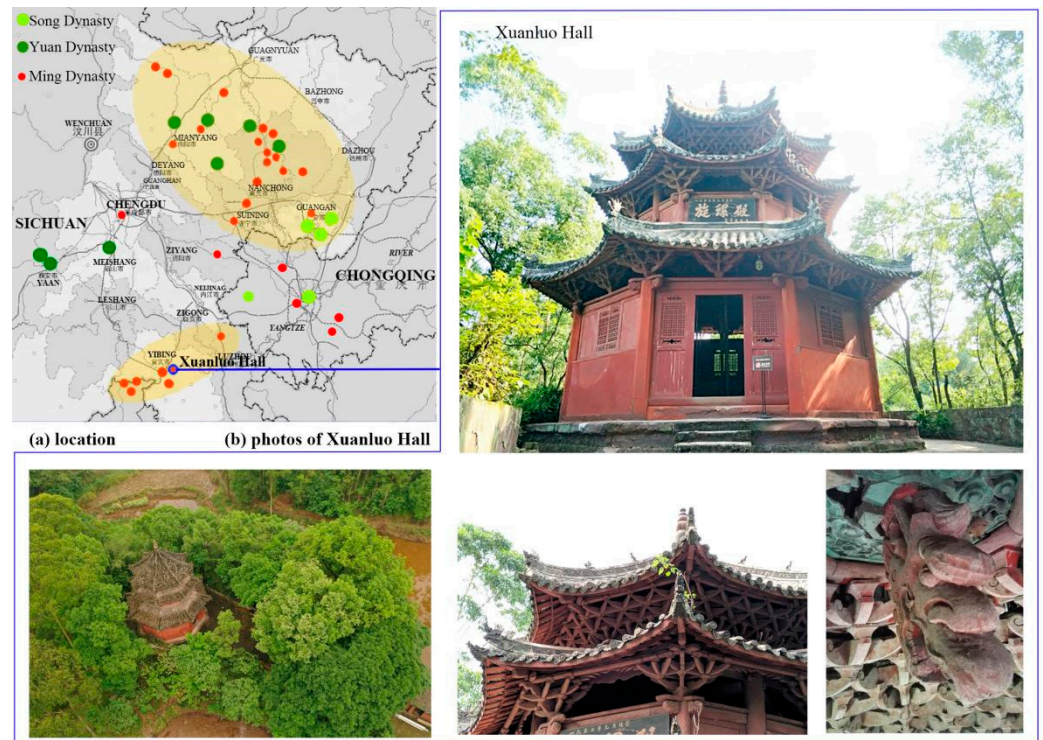
Figure 3. Study site: (a) Location; (b) The photos of Xuanluo Hall.
