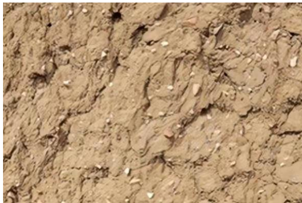
Figure 22. The rammed earth wall.
