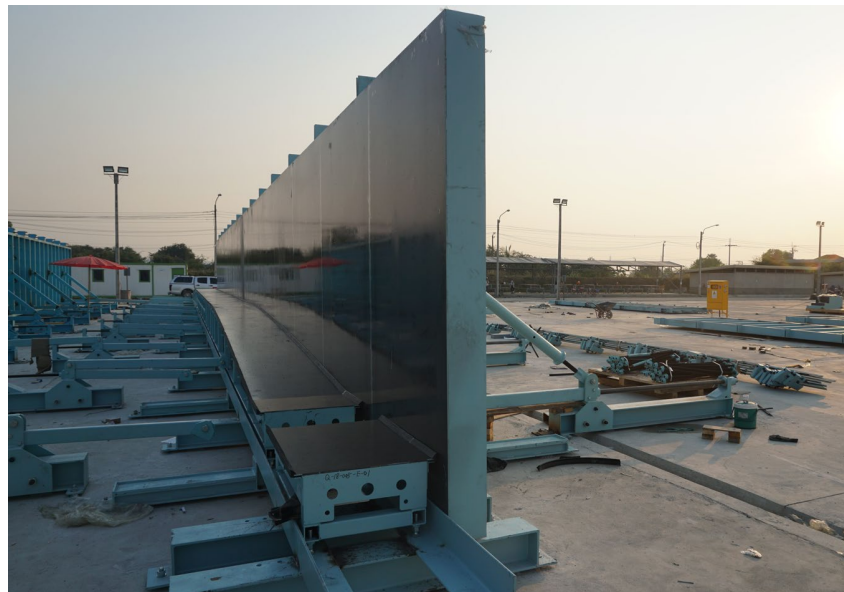
Figure 5. Typical view of formwork.
