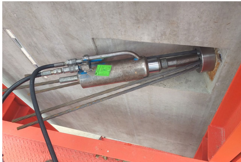
Figure 4. Application of tension to the PT tendons.
