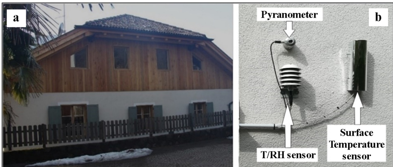
Figure 4. (a) Northeast wall monitored. (b) External sensors installed (Pyranometer, T/RH sensor, Surface temperature sensor).
