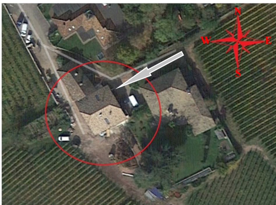
Figure 2. Plan overview of the analyzed building. The location of the wall that was examined for this study is indicated by the arrow.
