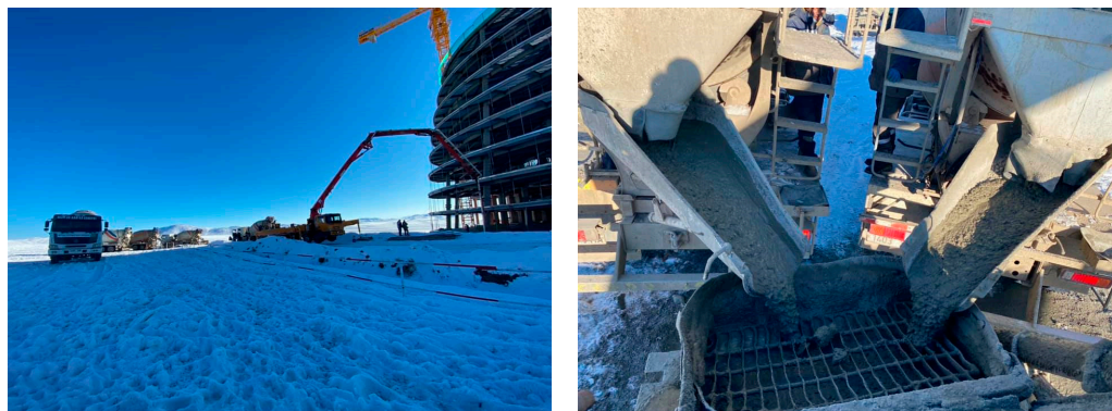
Figure 3. Construction site in December 2020 (average temperature was -17.7\text{ }^{\circ}\text{C} ).
