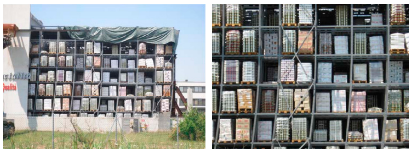
Figure 4. Seismic deformations of steel scaffolding systems [1].
