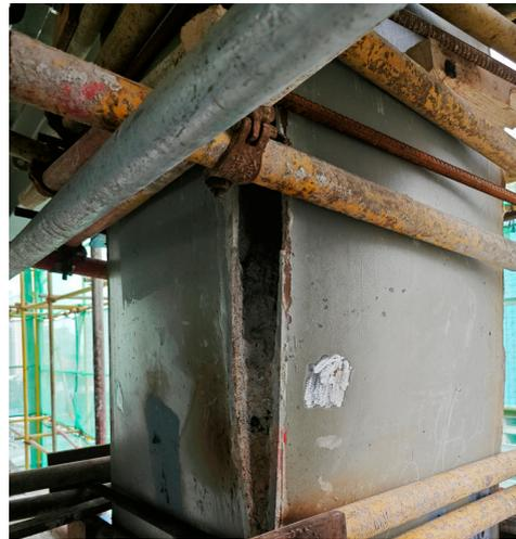
**Figure 1.** Welding joint failure of CFST column during concrete casting.
