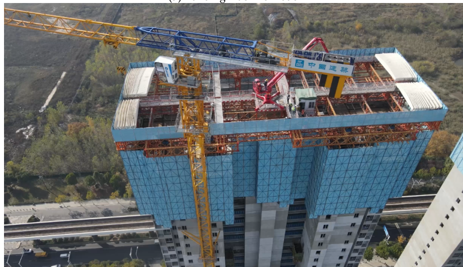
(b) Building machine live scene
