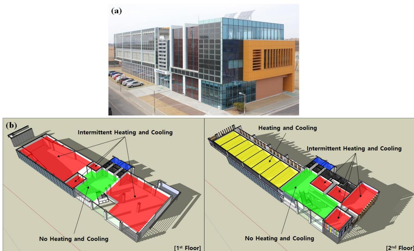
**Figure 1.** (a) Exterior of the Global Environment Research (GER) building; (b) spatial compositions and heating and cooling patterns of the first and second floors.
