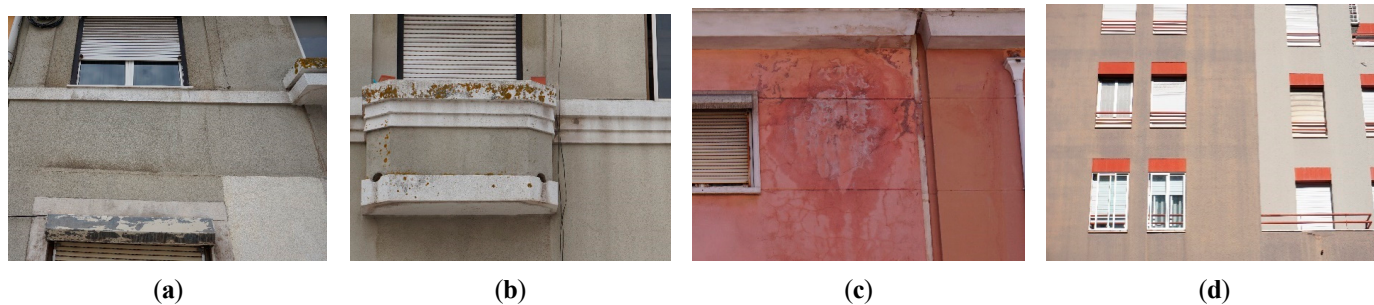
Figure 2. Different types of stains: dirt (a), biological growth (b), efflorescence (c), and discolouration (d).
