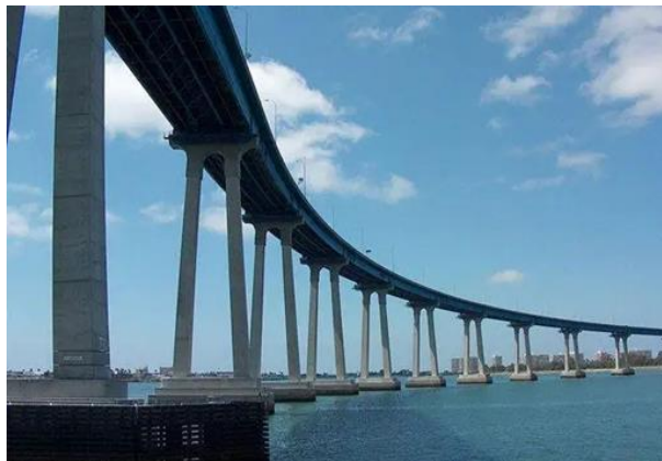
Figure 2. Curve-type approach bridge across the sea.
