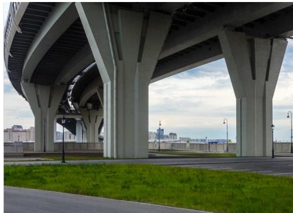
Figure 1. Curved crossing bridge.
