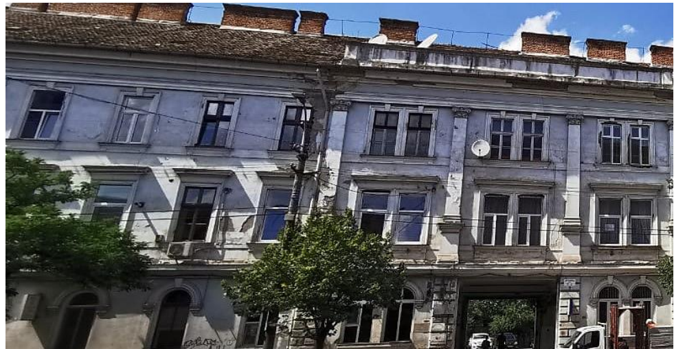
Figure 5. Facade to be rehabilitated.
