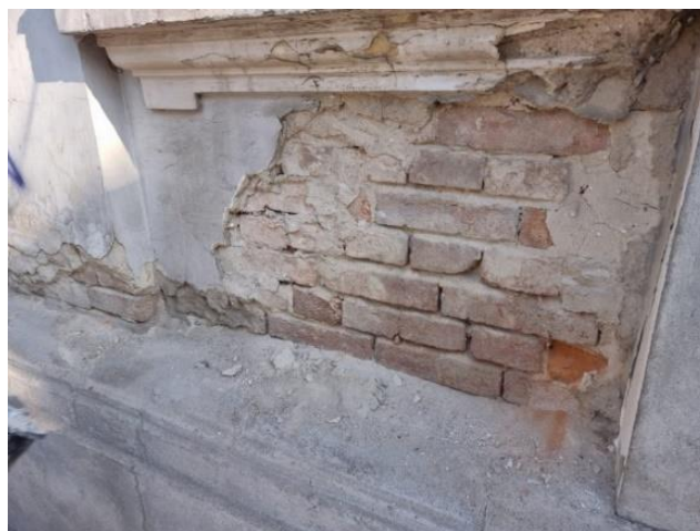
Figure 4. Plaster waste gathering from the brick support layer.
