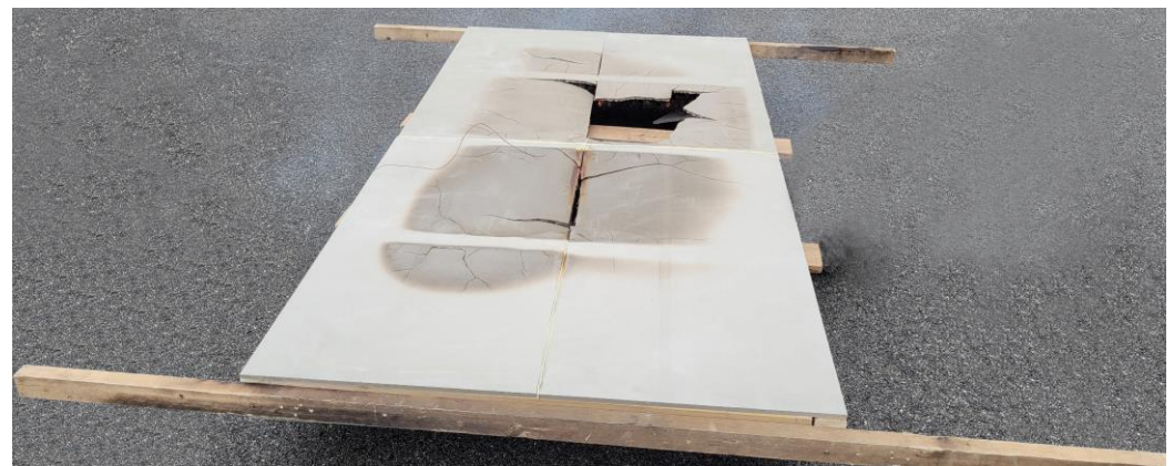
Figure 12. The condition of the structure after the test.
