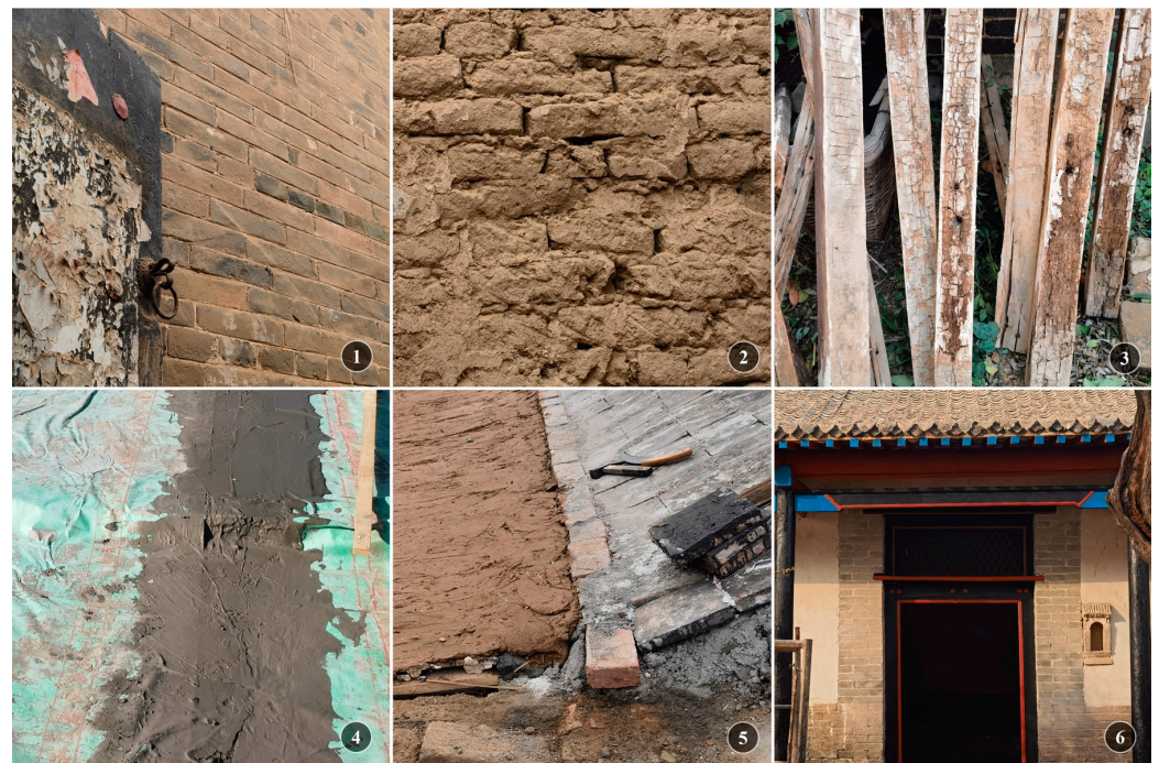
Figure 12. Materials for courtyard-style Confucian architecture: 1—green bricks, 2—wall blanks, 3—Larchwood, 4—JS waterproof layer, 5—thatched back (ShanBei), 6—painted finishes. Photo by W. Rong.
