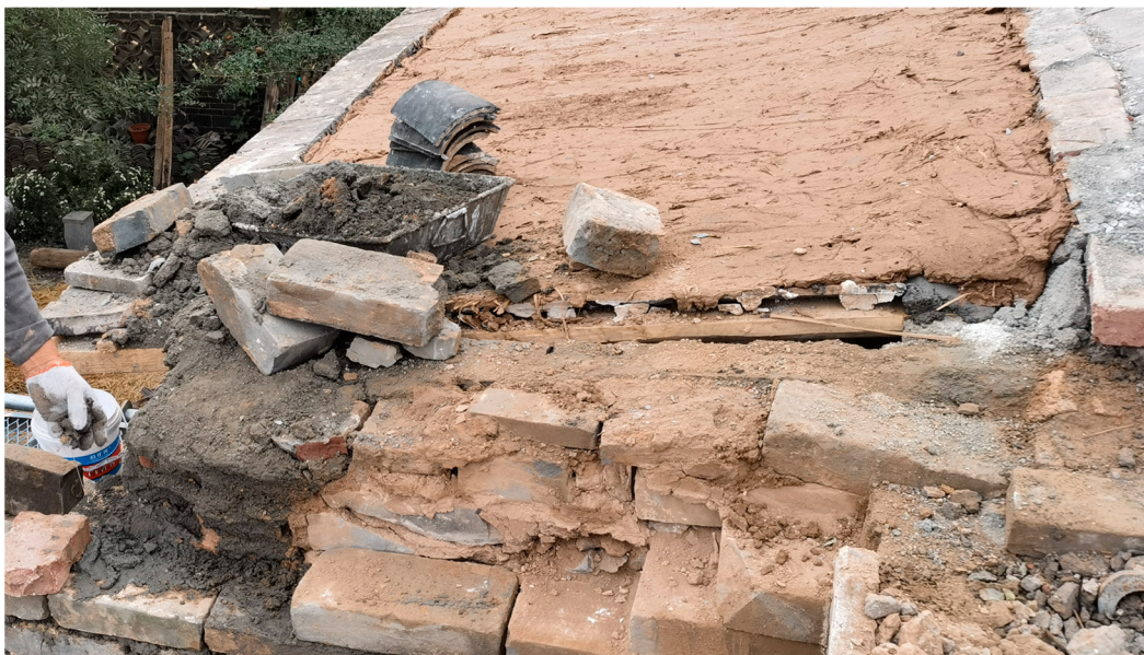
Figure 13. Thatch back (ShanBei) construction process. Photo by W. Rong.
