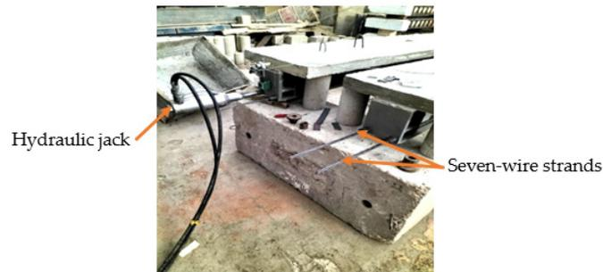
**Figure 4.** The application of the prestressing force.
