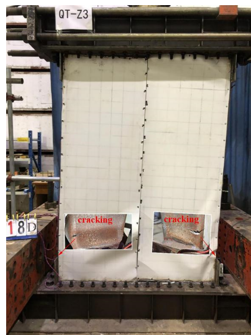
Figure 12. Failure image of QT-Z3.
