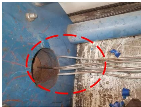
Figure 11. Breakage of strand at the fixed end.
