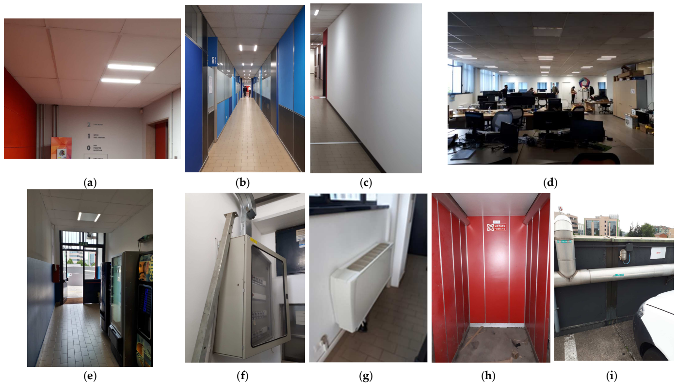
Figure 8. Examples of nonstructural elements of the case study building: (a) false ceilings with lighting elements X; (b) aluminum-glass partitions; (c) drywall partitions; (d) office furniture; (e) vending machines; (f) electrical cabinets; (g) fan coils; (h) elevator; (i) piping system.
