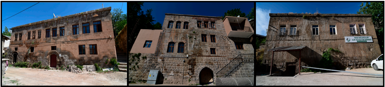
Figure 17. Some examined masonry structures.
