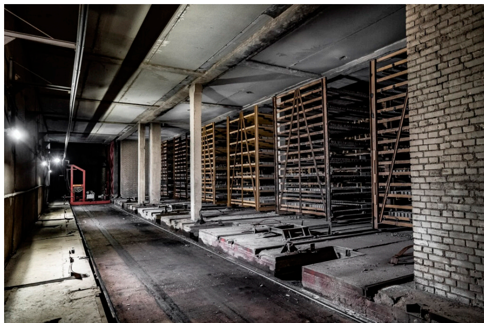
Figure 7. Stacking products on drying trolleys.
