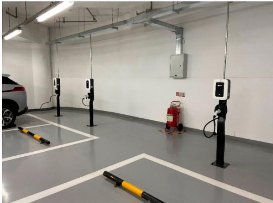
**Figure 3.** Realistic representation of the installation of EV charging piles.
