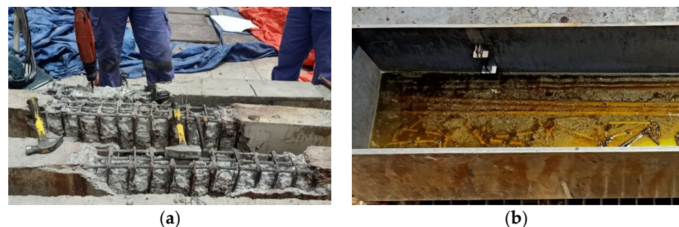
Figure 8. Extraction of corroded bars and rust removal: (a) extraction of steel coupons; (b) corroded bars during chemical cleaning.
